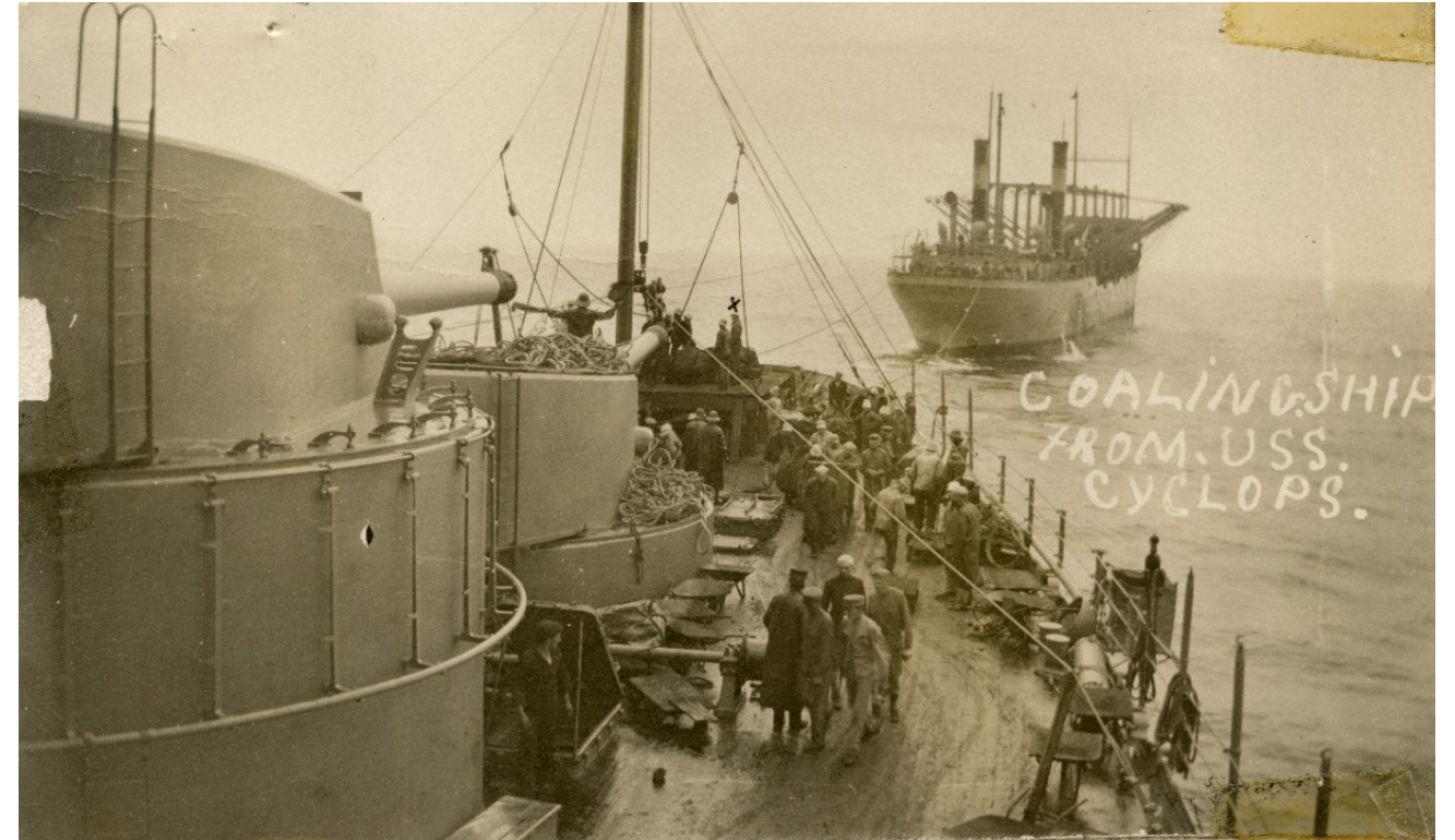
Battleship maneuvering to receive coal from USS Cyclops (Fuel Ship No 4). (U.S. Navy photo)
